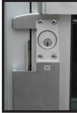
Close door and ensure proper alignment of lock.
