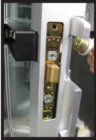
Replace lock into door.
